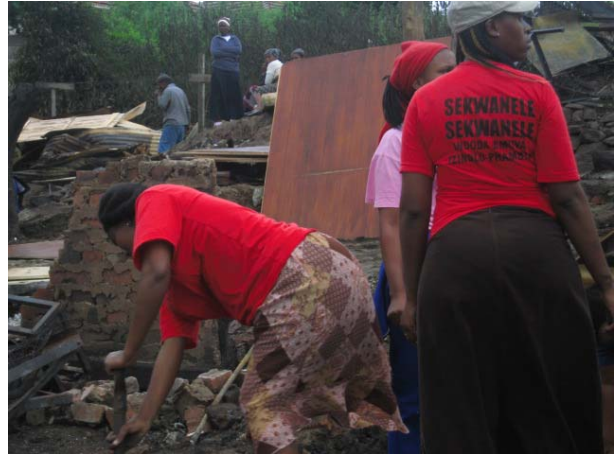
Abahlali working to rebuild Lacey Road
